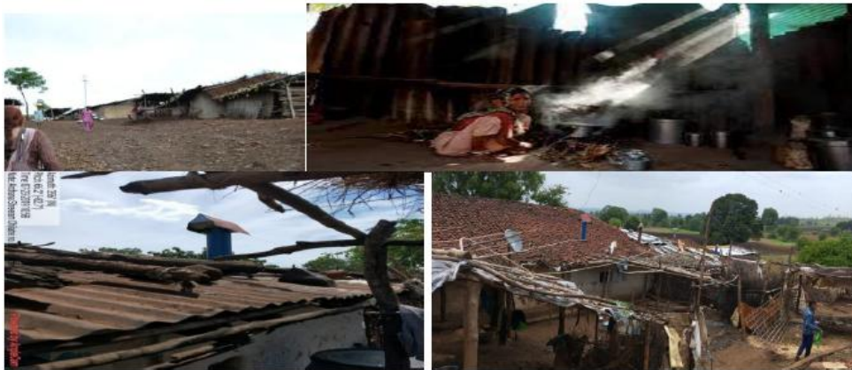
Fig 1. Village huts with smoke
